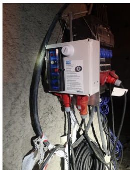
Figure 10. The Anybus Wireless Bolt LTE attached to the control unit
